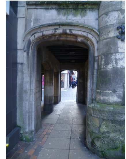
Plate 18 The passageway through the Stonebow and Guidhall building, High Street
