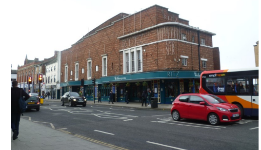
Plate 60 Former Ritz cinema, High St is a building of local interest dated 1937 and has unique external neon lighting
