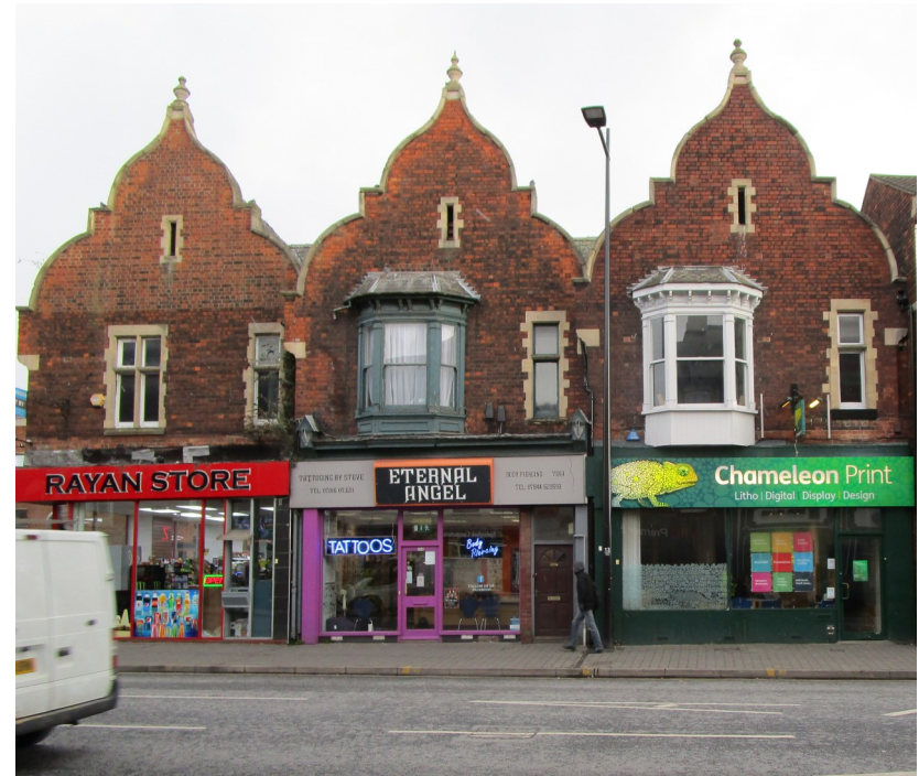
Plate 76 No. 365-367 High St, the contribution of these buildings of local interest to the conservation area is undermined by the over large fascia signs, use of modern materials, internal illumination, and the lack of proportions and detail of a traditional shop front, including pilasters and stallrisers. The palette of colours could be improved to better reflect the historic character of the area.
