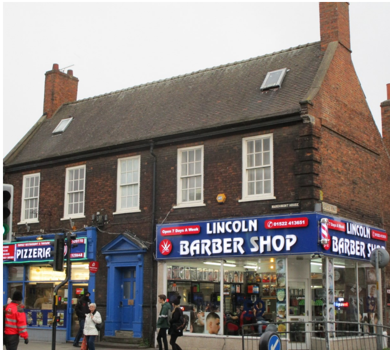
Plate 75 No. 363-364 High St, the historic interest of this listed building is considerably undermined by the over large fascia, use of acrylic and internally illuminated signage.
