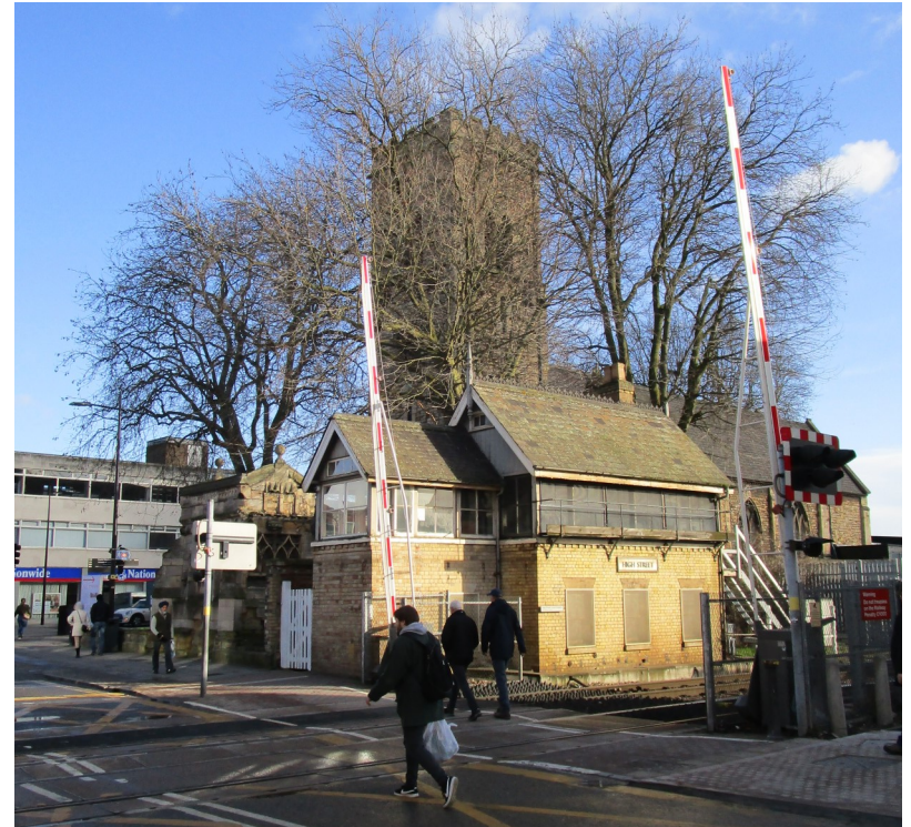
Plate 58 Railway signal box, High St is a Grade II listed building and is an early and largely intact example of a GNR signal box, dating from 1874.
