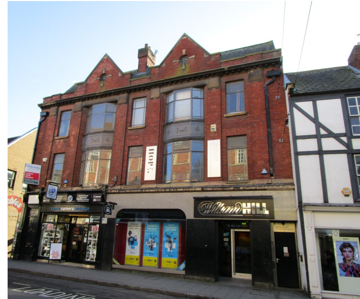
Plate 65 No. 4 Silver St is early C20th and has distinctive canted bay windows with decorative metal infill panels and brick pilasters.
