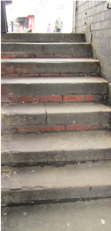
Plate 26 Stone and brick steps leading from west side of High Bridge to the river
