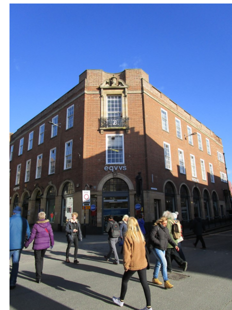
Plate 16 No. 280-281 High Street and 1-3 Clasketgate, Former Boots Department Store and Job Centre
