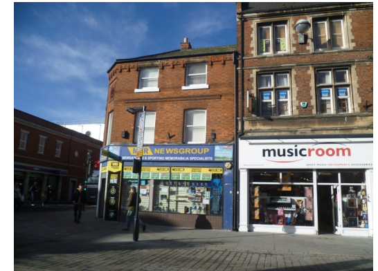
Plate 15 No. 159-162 High Street, purpose built commercial buildings
