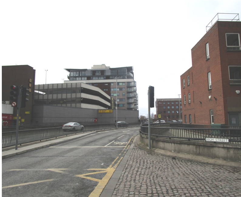
Plate 69 The construction of Wigford way has cut through the historic burgage plot development here and created an open, highway-dominated space at odds with the historic character here.
