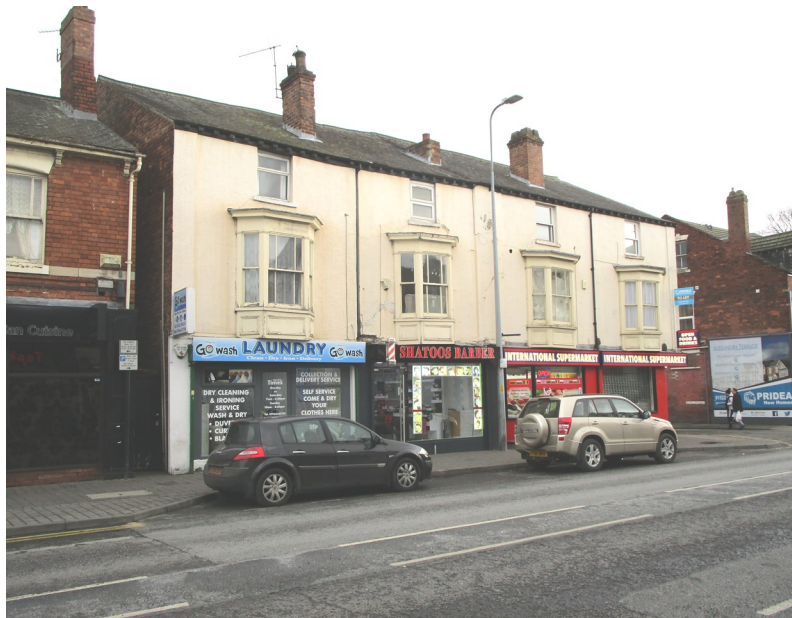
Plate 79 No. 372-374 High St, whilst fascia are relatively small, they do not form part of a traditional shop front composition, and modern materials and internal illumination detract from the conservation area. Projecting signs are boxy and shutter housing on the left hand building makes the fascia boxy.
