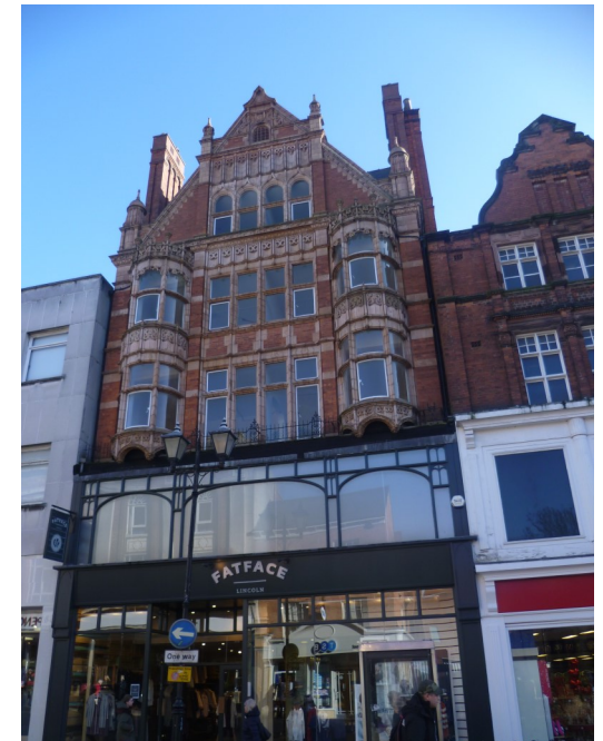
Plate 42 No. 305-306 High St shop and offices, dated 1900 is brick with terracotta dressings and a slate roof with 2 panelled side wall stacks. It is in the Flemish Renaissance Revival style and has giant pilasters, domed finials, an enriched moulded cornice and coped gable.
